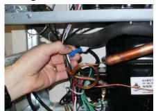
Next, insert end of tube into fitting.
