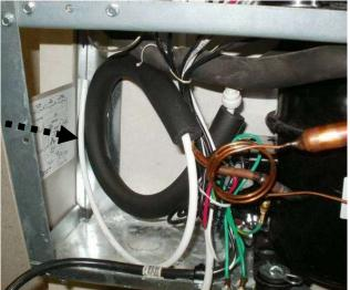
For <u>split level</u> "Versafiller ready" coolers, the tube to plumb in the Versafiller is packaged in the dummy unit or found inside the Bottle Filler.
