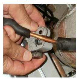
Install TEE fitting by connecting the copper tubing to each end. Then install the 32" piece of plastic tubing to the TEE branch.
